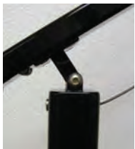
Pivoting top rail attachment
